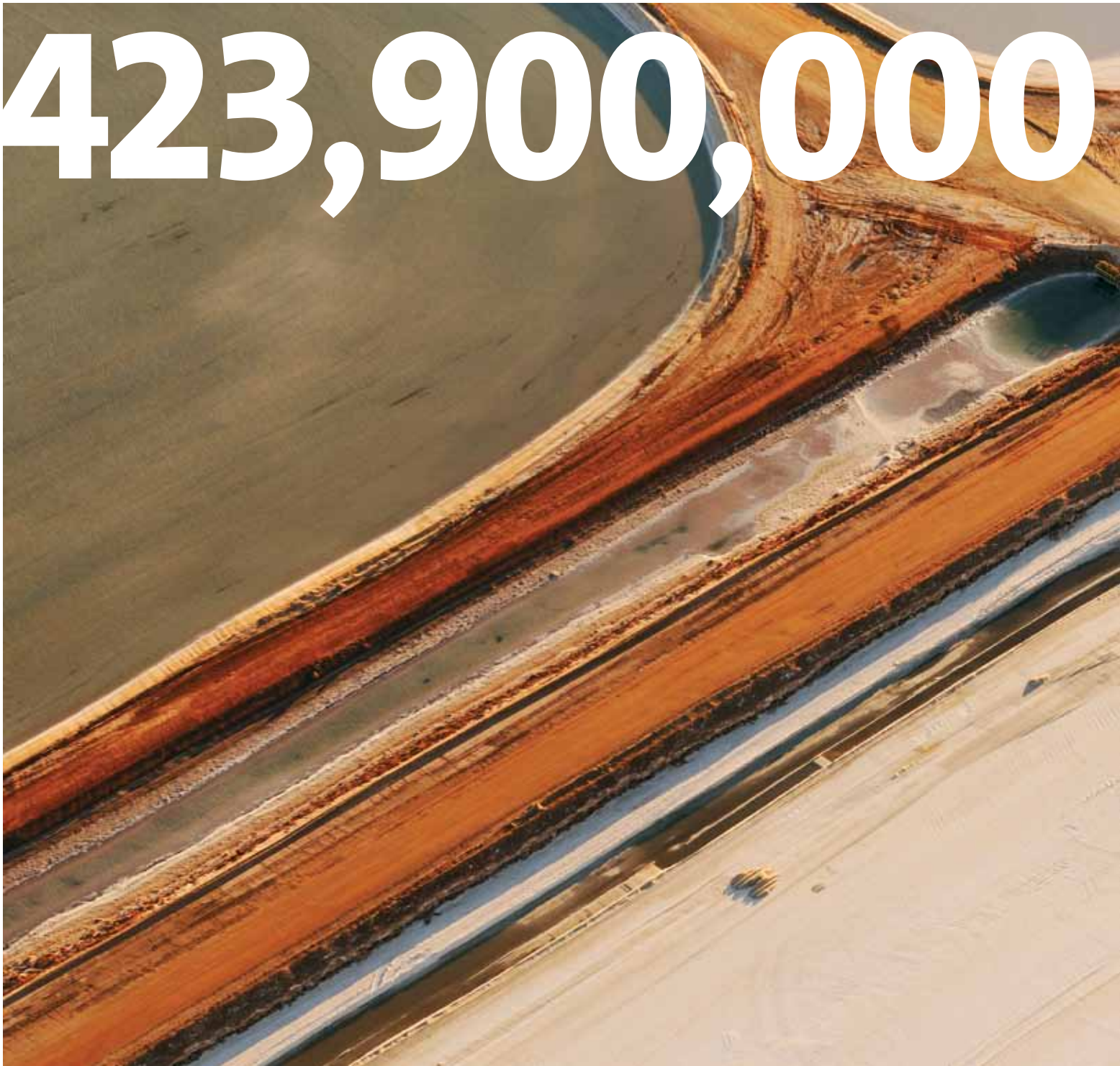
Aerial of Salt production works, Port Hedland, Western Australia.
